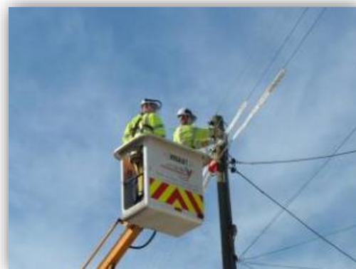
Fitting low energy LED lamps
