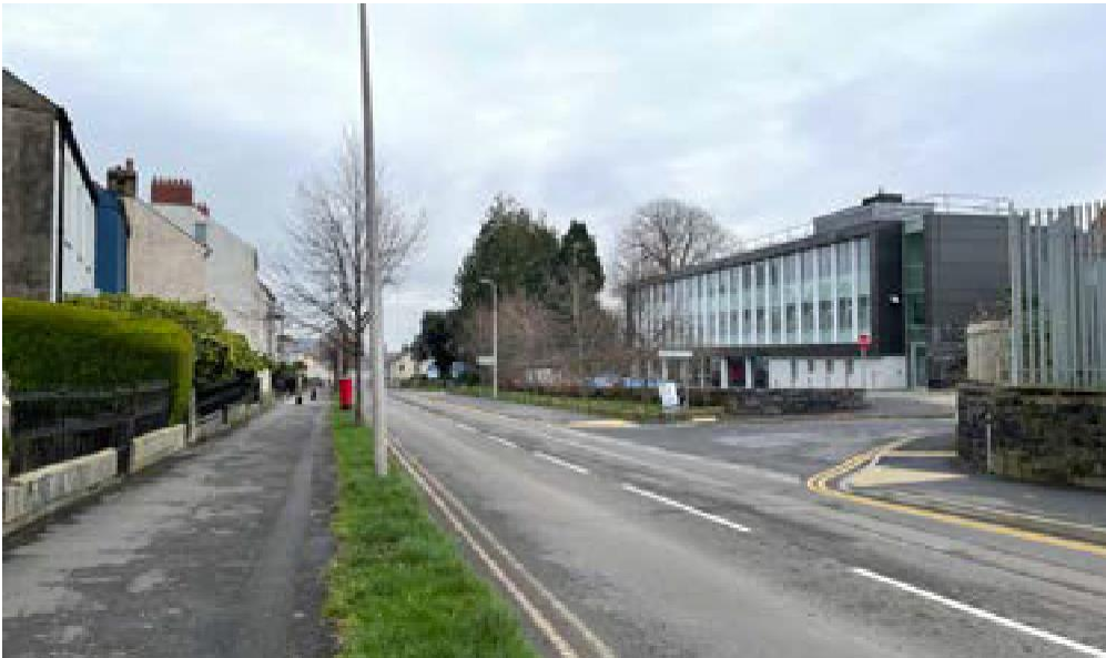
Contemporary development in Picton Terrace Conservation Area which may be considered of good design but which does not sit comfortably in the streetscape
