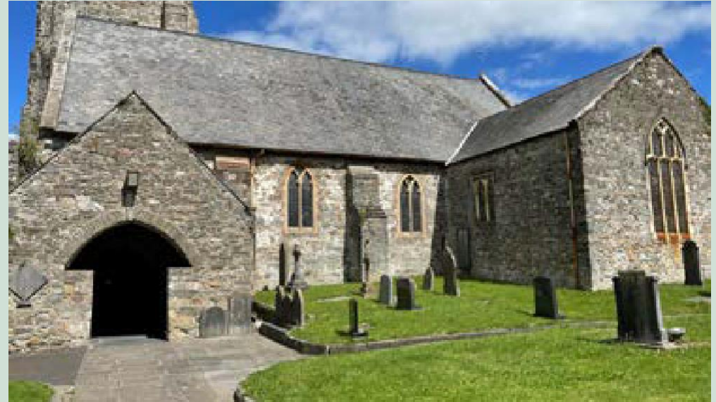
Intangible elements - The uses of buildings such as churches and churchyards retain links to the people and events which have come before
