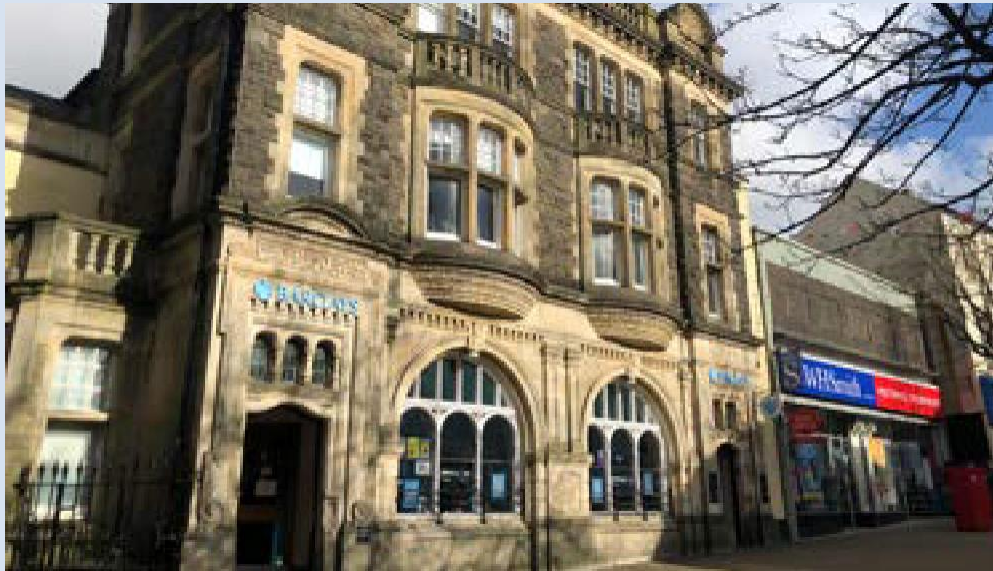
Aesthetic Value - This can be a subjective value to assess, but generally buildings of high aesthetic value will share aspects such as high quality materials and architectural details
