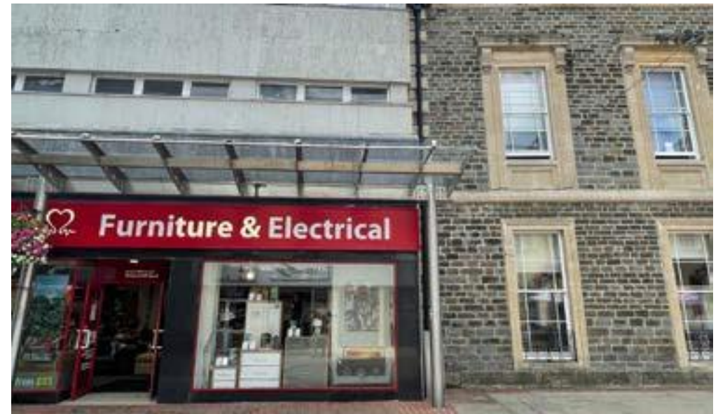
An example of insensitive late 20th Century development next to the Grade II listed Llanelli central library
