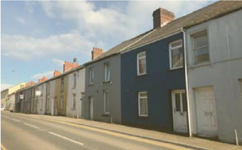
Former burgage plots recognized through the narrow frontages. The terrace provides consistency in building width, height and relationship to the street edge
