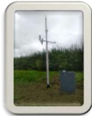
Sensors installed at the outstations store and relay information on air and road surface temperatures, dew point, wind speed and direction, and presence of salt. The information is interrogated by computer via a web bureau service. All the weather stations now include cameras to provide live images (excluding Black Mountain site which is solar powered)
