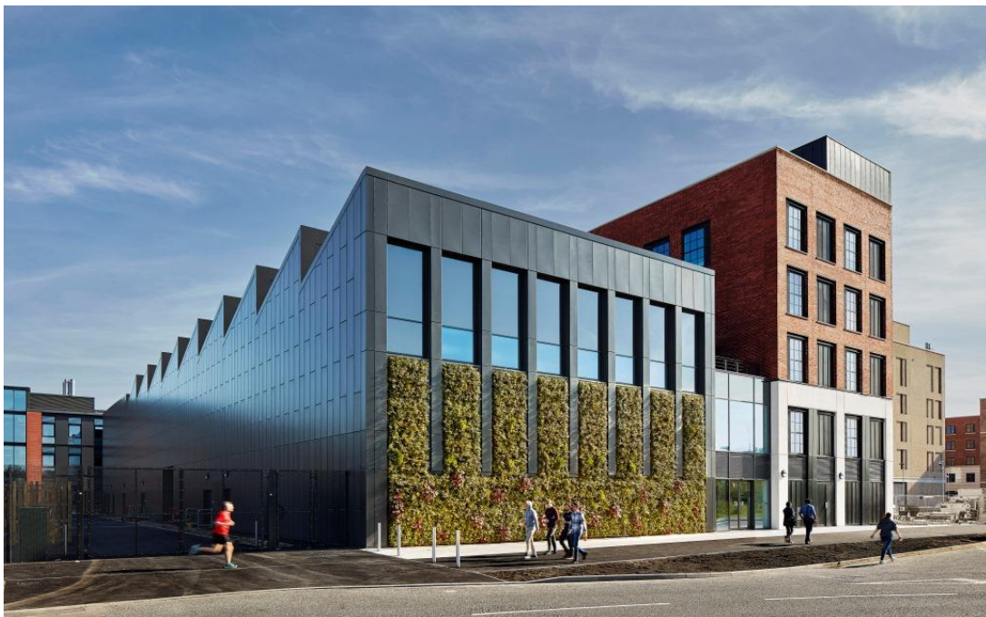
Picture: the outside of the IMPACT building, which features a giant living wall with over 5,000 plants (Image courtesy of AHR)
