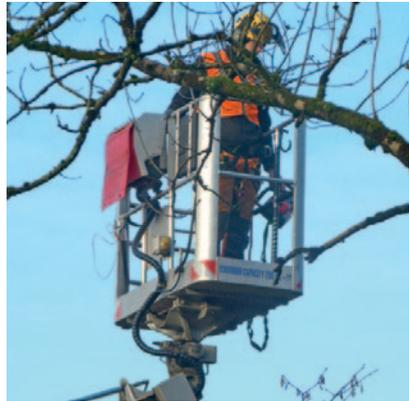
*Many trees with ash dieback will be unsafe to climb and will have to be felled using elevated platforms*
