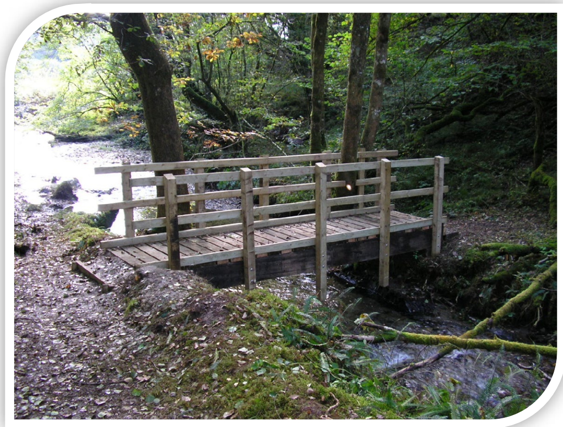
Timber Footbridge, Cilycwm
