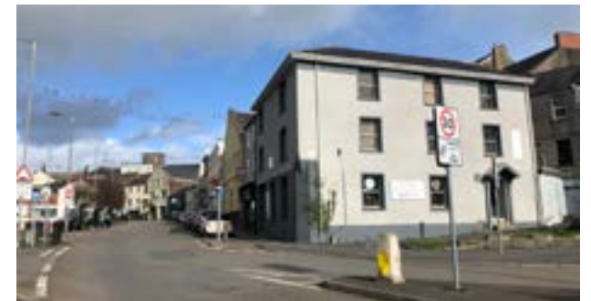
Southern entrance to Blue Street
