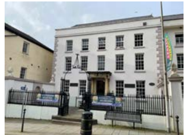
Metal railings to Carmarthen library
