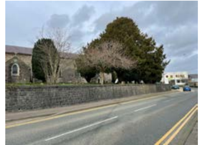
Stone boundary wall to St Peters Church
