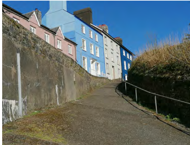
Chipped tarmac to Bank Buildings
