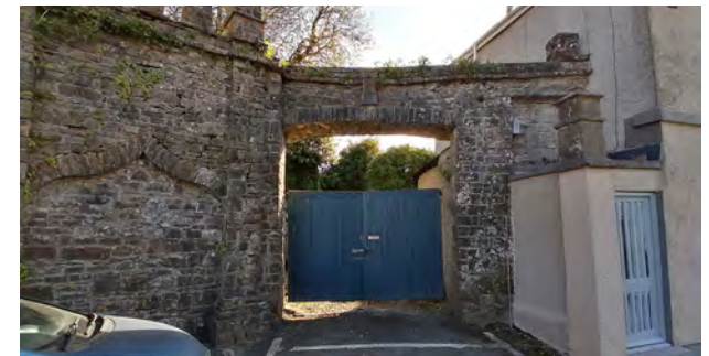
Crenelated masonry wall to Abbey Terrace
