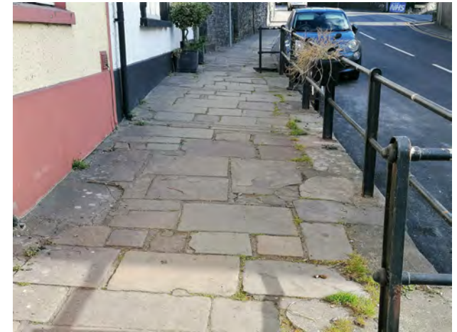
Stone slabs to Bridge Street
