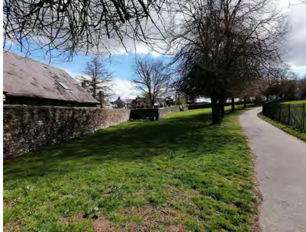
Rubble stone wall and open metal fencing
