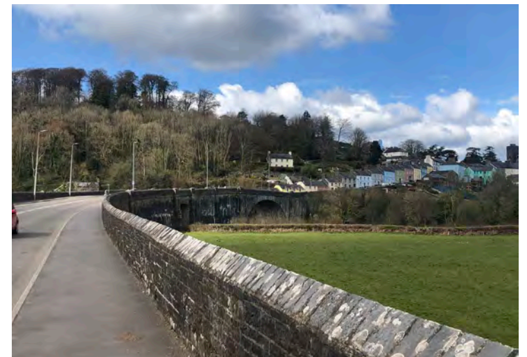
Llandeilo Bridge looking towards Bridge Street
