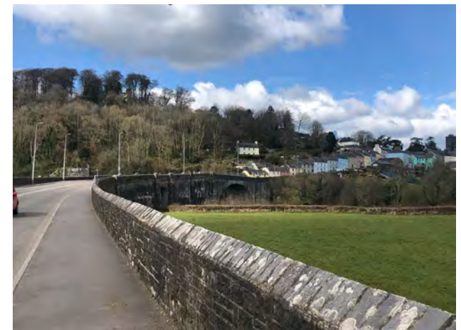
Southern entrance into the CA looking towards Bridge Street
