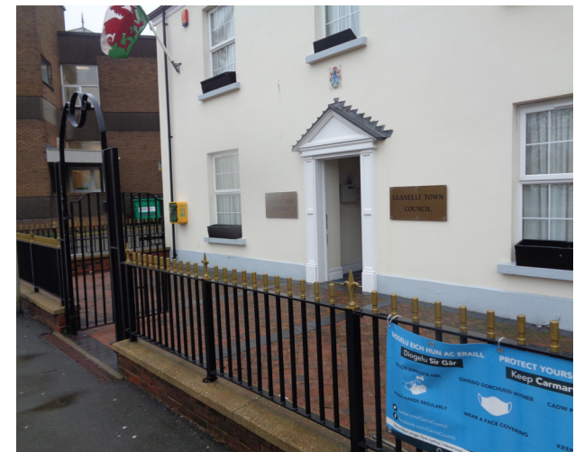
Metal railings at the Old Vicarage
