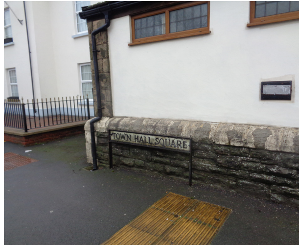
Front boundary wall to the community hall with infill development behind
