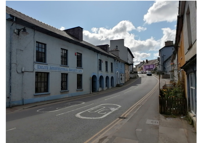
View north along Bridge Street
