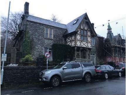
Building facing Market Hall building (former National school), Carmarthen Street
