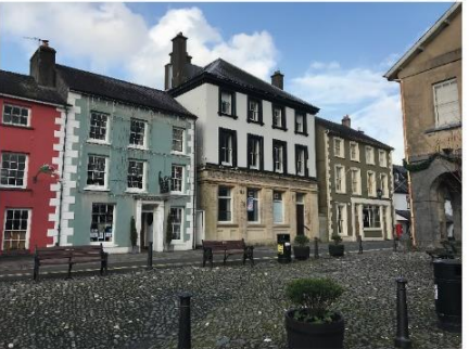
Street frontage at Market Square
