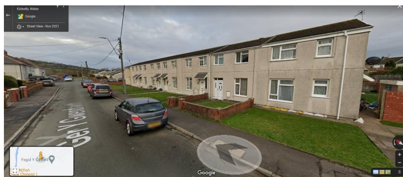
Figure 37 – Photo of the properties at Ger Y Gwendraeth that were flooded.
