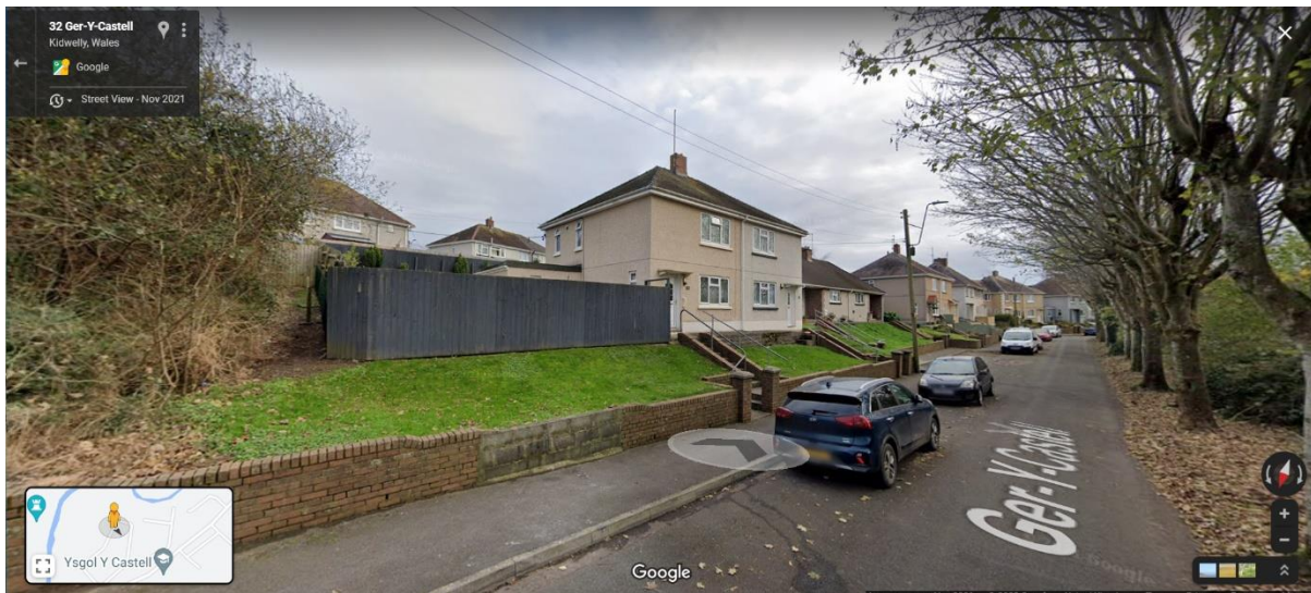
Figure 38 – Photo of 32 Ger Y Castell that had internal flooding from the rear.
