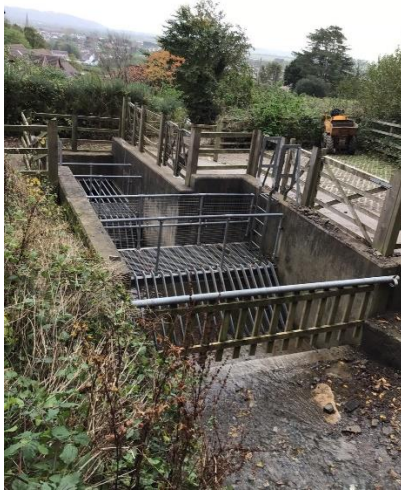
Figure 30 – On the left, the new trash screen as seen today, on the right, the screen that was replaced in 2014.
