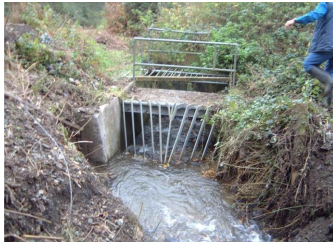
Figure 30 – On the left, the new trash screen as seen today, on the right, the screen that was replaced in 2014.
