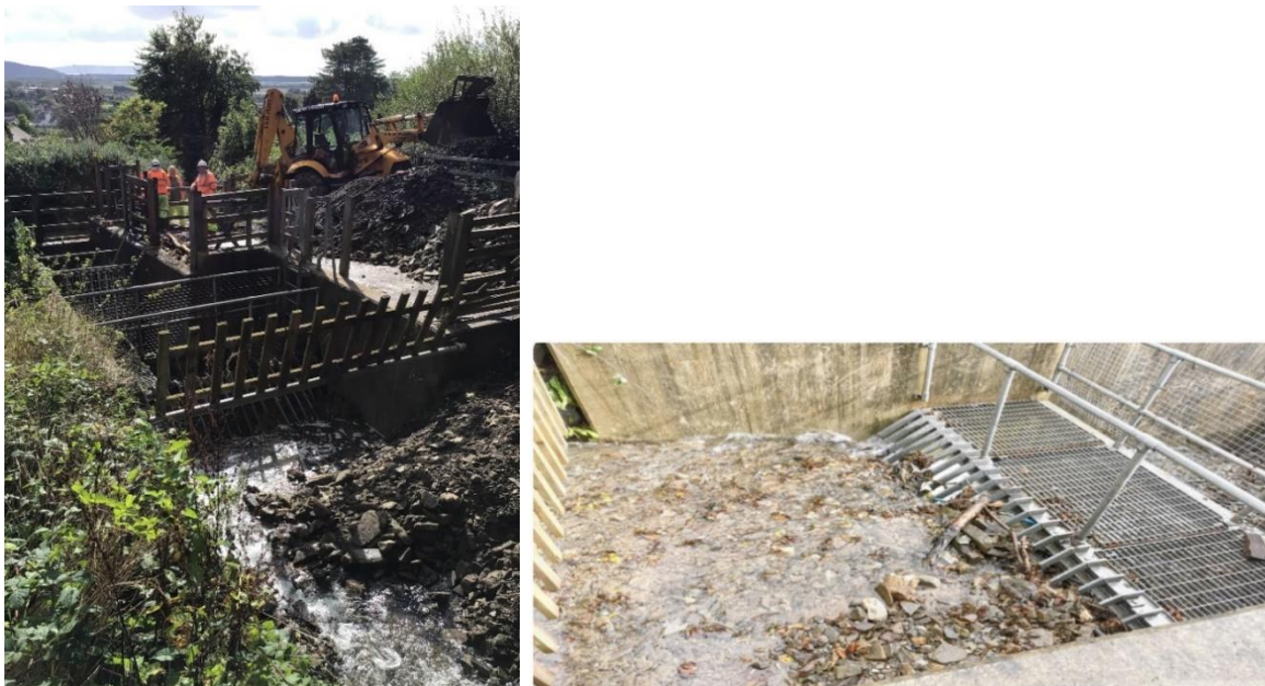
Figure 22 - Photos of the debris removed after the flooding event on the 4 th October 2021 at Cae Ffynnon.
