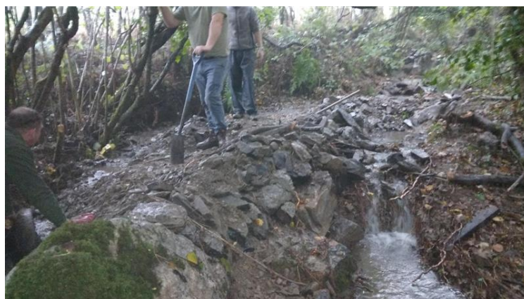
Figure 24 – Photo of Kidwelly residents unblocking the Cae Ffynnon watercourse north of Cae Ffynnon. In the picture, the water is flowing down the footpath, the watercourse is where the men are standing.
