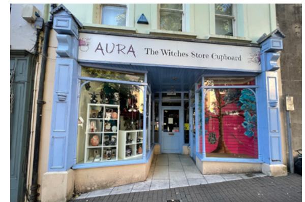
Mid 19th Century shopfront in Carmarthen.
