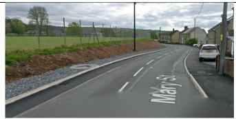
480m of upgraded footway along Heol Blaenhirwaun Road inclusive of new dropped kerbs and tactile crossing points.
