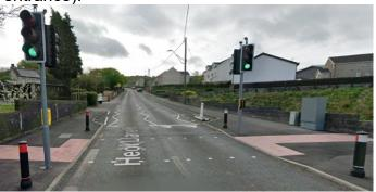
Installation of plateau crossing points at key points within the village to encourage active travel movements and reduce vehicle speeds.
