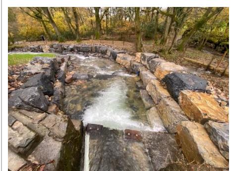
A technical fish pass easement at perched bridge on Afon Ceiliog near Llanybydder
